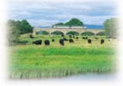
Train on Melling Viaduct
